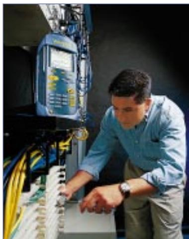
The LT 8155 is the perfect tool for certifying all cabling installations, plus measuring headroom and performance grading for enhanced cabling up to 155 MHz. Tests can be viewed in graphical plot format as well as text. 1,500 Autotest results can be stored resulting in enough capacity for several days testing.
